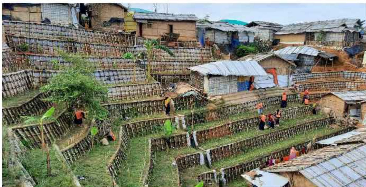
CFW participants working on slope stabilization in Ukhiya, Cox's Bazar, Bangladesh. © IOM 2023/Osman TAHER
